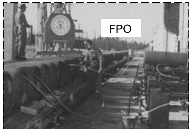
Fig. 2-32. Unloading mustard agent from 1-ton containers on flat cars at Pine Bluff Arsenal, Arkansas, in 1943. Apparently unloading and loading mustard agent were considered to constitute different hazards (see Figure 2-31). Note that the operator is wearing a face shield, apron, and gloves, but not a protective mask. Photograph: Chemical and Biological Defense Command Historical Research and Response Team, Aberdeen Proving Ground, Md.
